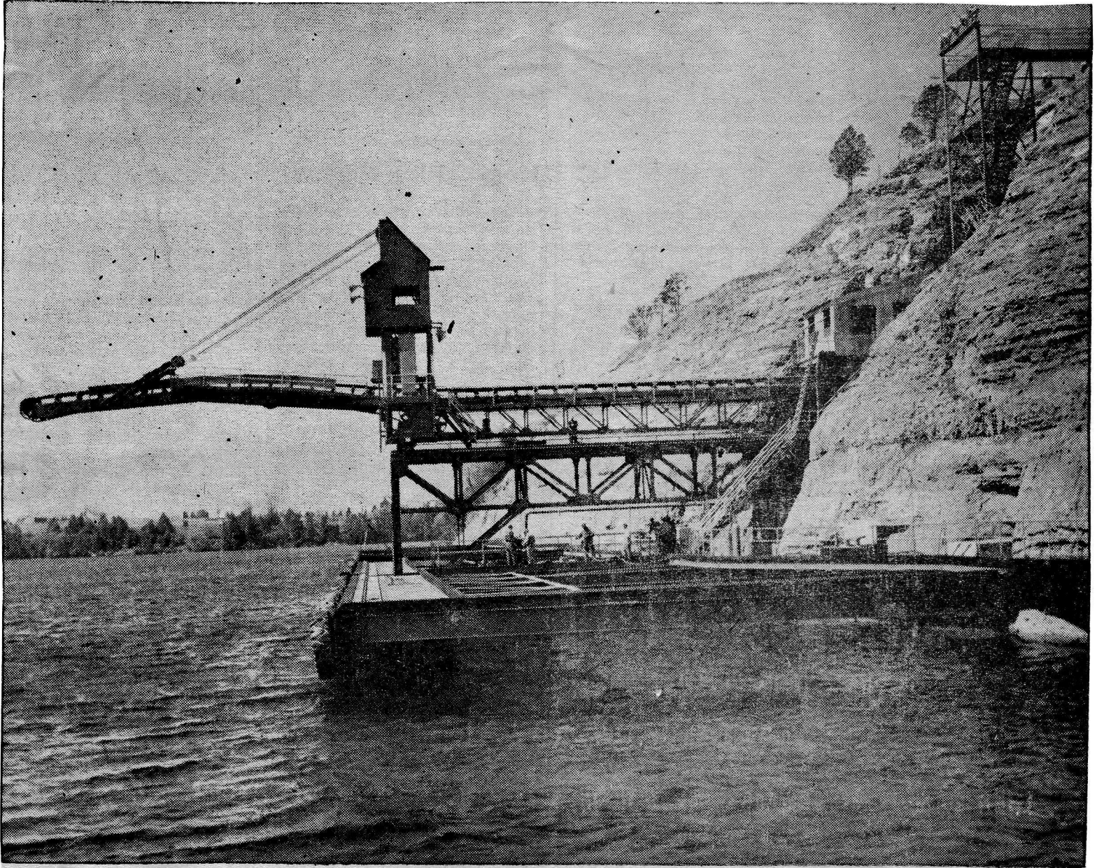
noraton Mining Company dock and rail to ship transfer facilities at the High Shore, Picton Harbour. The Hadgson Studio photo shows at bank and conveyor belt extension for feeding ore to boat. The first boat arrived Tuesday morning, May 10th.
