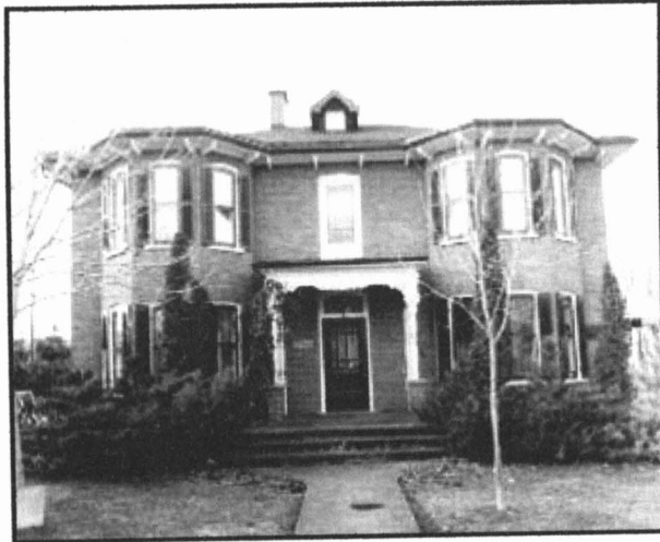
The Marmora Foundry "old company house" Renovated by George B. Bleecker in 1887
