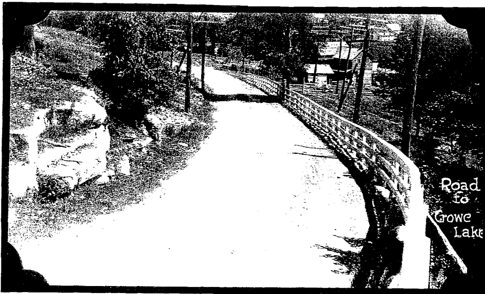
Road to Crowe Lake before #7 was constructed
