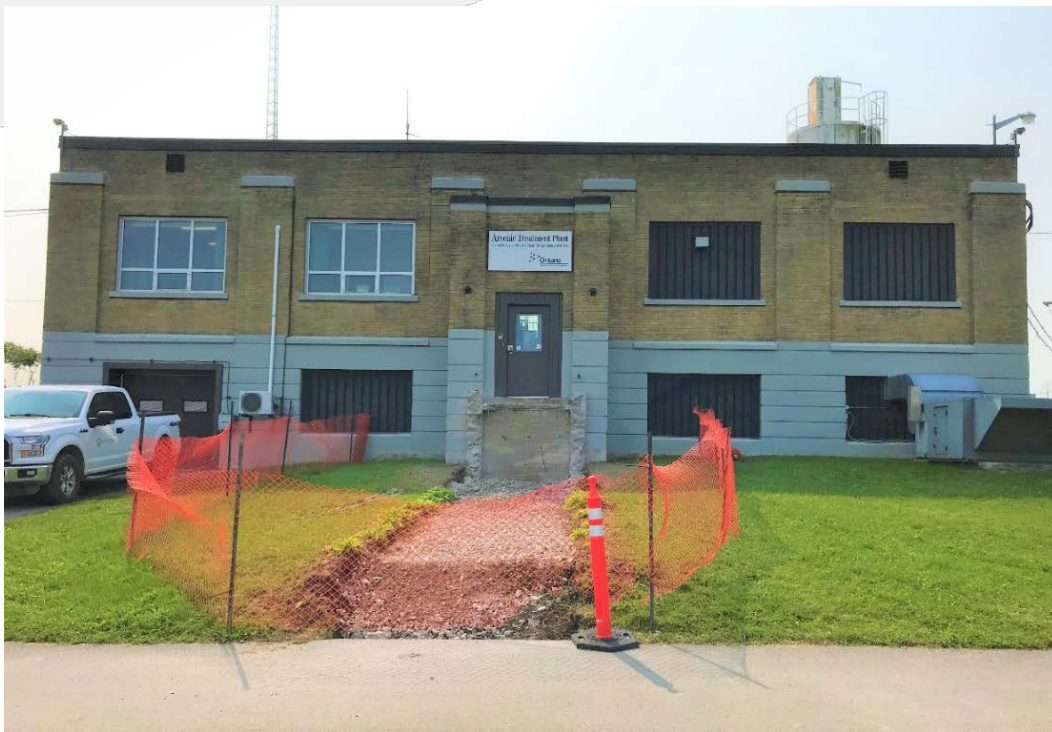
Photo of Arsenic Treatment Plant undergoing outside maintenance.
